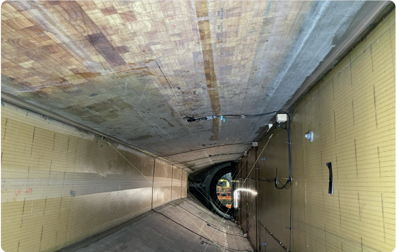
Figure 2 - String-potentiometer instrumentation is installed inside the blade box section at a measurement station.
