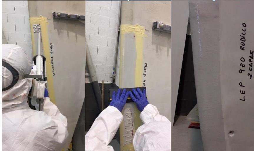
Figure 52 - AHP LEP Service System application (Siemens Gamesa service).
