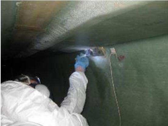
Figure 122 – Installation of X-Stiffener in 15m section
