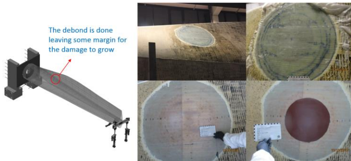
Figure 39: Debonded skin setup in SSP34 blade installed at DTU. On the right, a detail of the defect manufacturing highlighting the size of the defect introduced.
