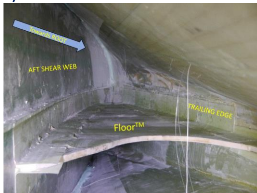
Figure 2: A) The Bladena Floor™ technology works as a horizontal shear web installed between the aft shear web and the trailing edge on the Root-Transition zone of a wind turbine blade. B) Floor™ is retrofitted in an SSP34m blade. It can be seen how the aft shear web spans out and connects with the trailing edge/blade root. C) Floor™ is retrofitted in an LM58.7m blade. The retrofitted Floors™ in the SSP34m blade and the LM58.7m blade are used for demonstration purposes in the RATZ project [4] [5] [6].
