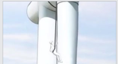
2. Access the turbine using rope or a basket
